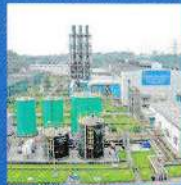
Dutch Bangla Power & Associates Ltd.
