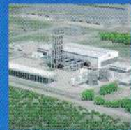
Orion Power Sonargaon Ltd.
