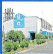
Orion Power Meghnaghat Ltd.
